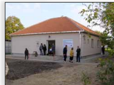
Busenje Educational Centre after the reconstruction
