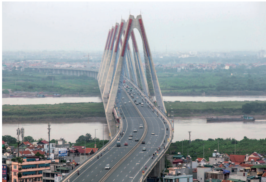
The completed Nhật Tân Bridge (Vietnam-Japan Friendship Bridge) in Viet Nam. The bridge will alleviate congestion and improve traffic efficiency across the Hong River in Ha Noi City and contribute to the city's economic development. (Photo: Shinichi Kuno / JICA)
