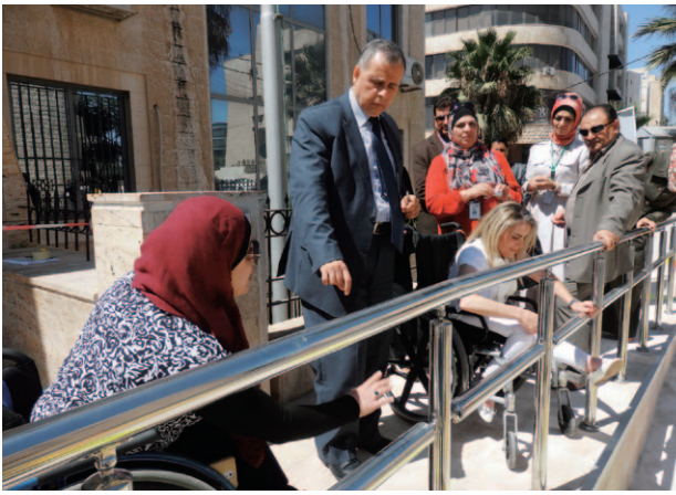
Improvement of a barrier-free environment is important for supporting the employment of people with disabilities in Amman, the capital of Jordan. The conditions on the angles of slopes, materials and handrails on the way to the Ministry of Labor in Jordan were improved by support from Japan. (Photo: Yahoko Asai / JICA Expert)
