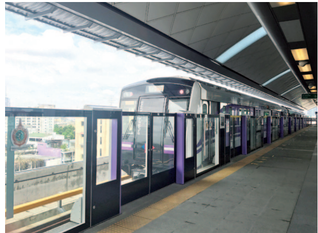
The Mass Transit System Project in Bangkok, Thailand. The railway which started service in August 2016 has an overall length of 23km, and adopted the first-ever Japanese railcars used in Thailand. (Photo: JICA)
