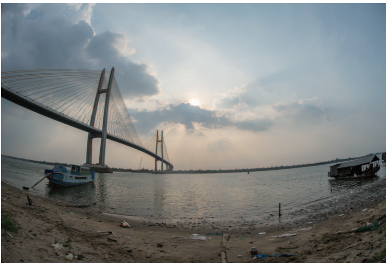
The Neak Loeung Bridge (Tsubasa Bridge) in Cambodia was opened to traffic in April 2015. The primary span is 640m with a total bridge length of 2,215m, and reaches 5,400m when including connected roads. Previously, crossing the Mekong River by ferry took one hour, but it has been reduced to approximately 5 minutes with the opening of the bridge. (Photo: Shinichi Kuno / JICA)
