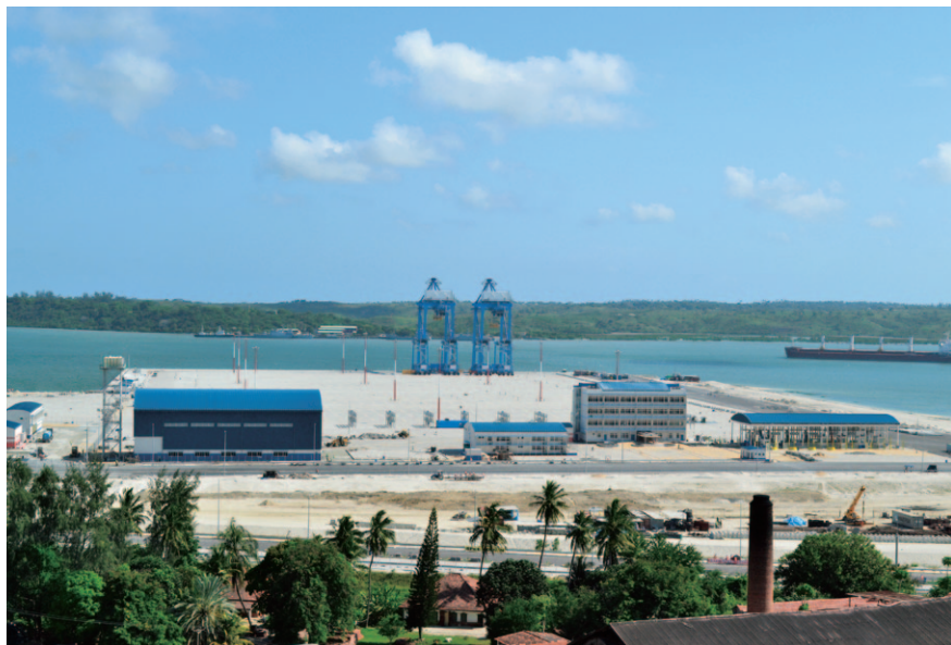
Mombasa Port, the largest commercial port in East Africa. It is the sole international trade port in Kenya, and also serves as a critical gateway port for inland countries of Africa such as Uganda and Rwanda. (Photo: Toyo Construction Co., Ltd.)
