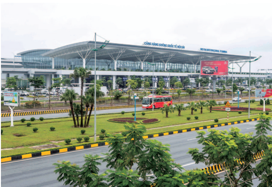
The Terminal 2 Passenger Building for international flights at Noi Bai International Airport, Viet Nam, which has large capacity for 10 million passengers (Photo: Shinichi Kuno / JICA)
