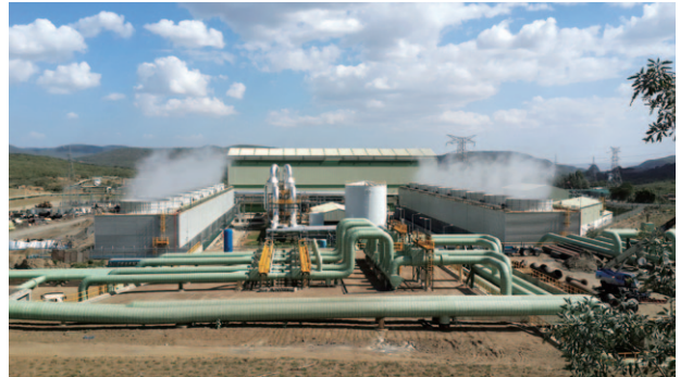
Attaining the improvement of stable supply of electricity in Kenya's Rift Valley Province through the construction of Units 4 and 5 of the Olkaria I Geothermal Power Station (70 MW × 2) (Photo: JICA)
