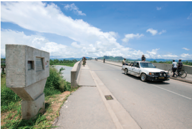
The Mangochi Road Bridge constructed with grant aid in Mangochi District in the southern region of Malawi. The bridge serves to invigorate the flow of goods through the Nacala Corridor. (Photo: Kenshiro Imamura / JICA)
