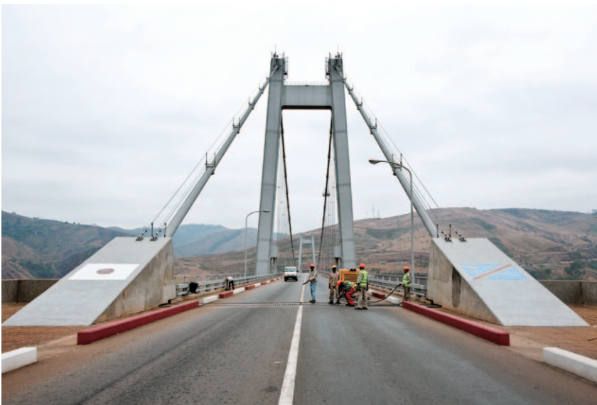
The Matadi Bridge, built with the assistance of Japan in 1983, is the only suspension bridge to cross the Congo River. Although regional conflicts began shortly after its completion, Japanese engineers were successful in transferring the related technologies, demonstrated by the bridge being well maintained for over 30 years since its completion. It is a symbol of friendship between Japan and the Democratic Republic of the Congo. (Photo: Shinichi Kuno / JICA)
