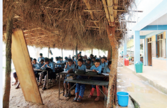
A lesson in a temporary classroom. School restoration work is underway in the background. (Photo: JICA)
