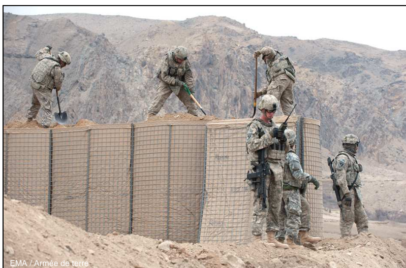
Figure 22 - Building a Bastion Wall in a Forward Operational Base (FOB).
